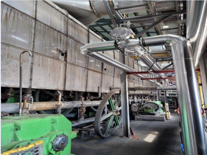
A Jetomat with its actuator at a dryer steam group
